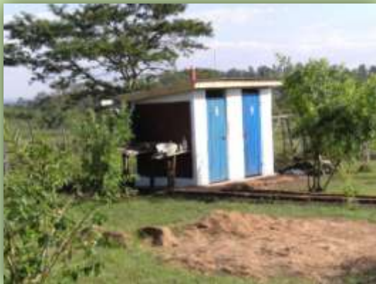
Gender segregated latrines at Karibuni.
